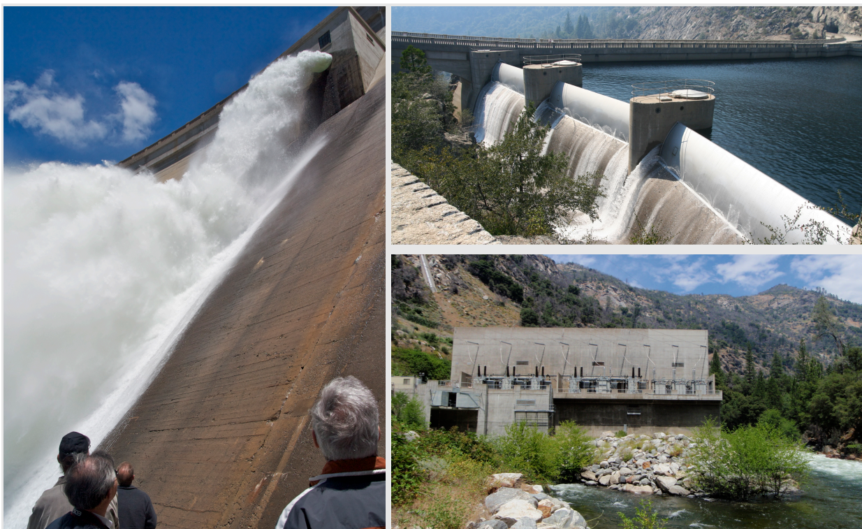
Figure 9. Selected project features in the Hetch Hetchy Reach: O'Shaughnessy Dam face valves (left photo); drum gates (top right photo); looking upstream at Kirkwood Powerhouse with the Tuolumne River to the far right (bottom right photo).
